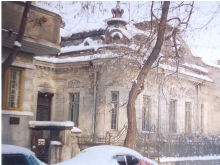
PHOTO 1. One of the many single storey houses constructed before World War I
