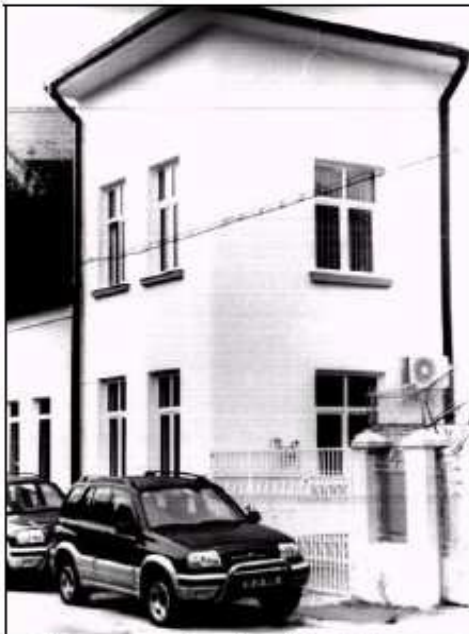
PHOTO 7. A former nationalized building, sold to tenants, then purchased by real-estate agents who turned it into office space
