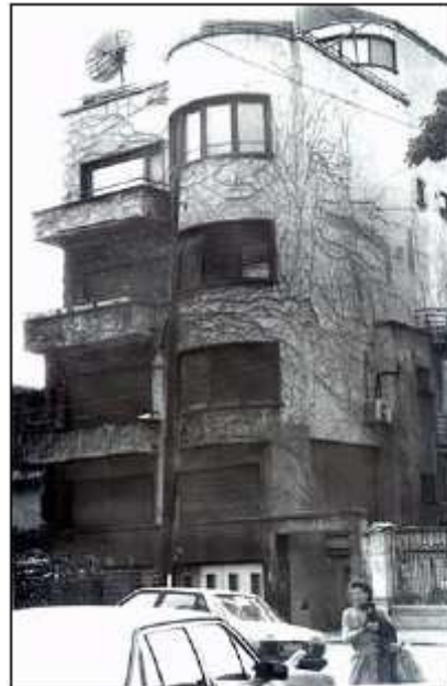
PHOTO 4. An apartment building built between World War I and World War II
